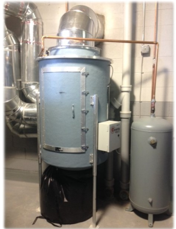
FRP filter w/ optional radius inspection door and compressed air storage tank
