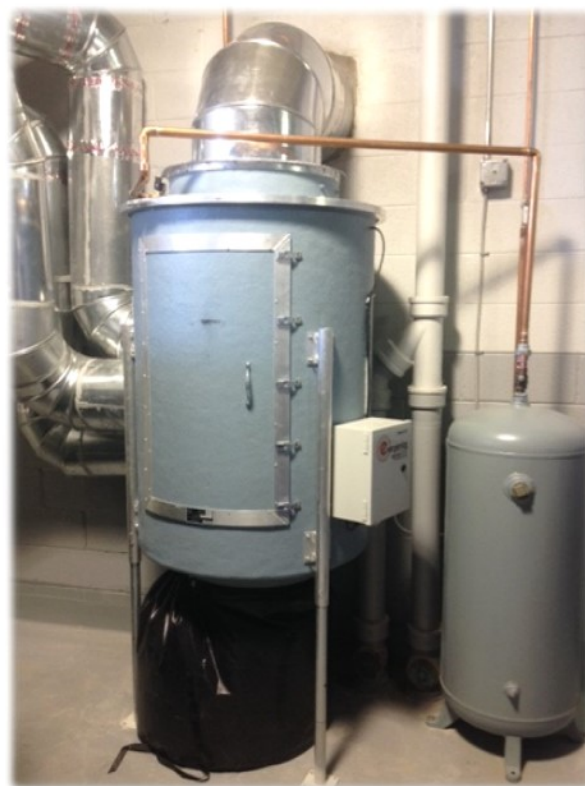
FRP filter w/ optional radius inspection door and compressed air storage tank
